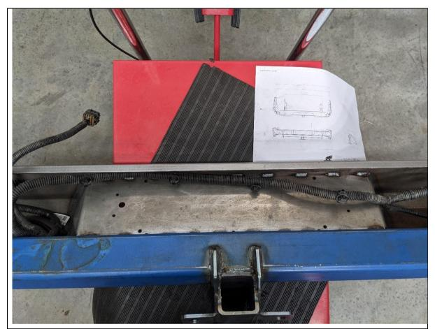
13. Fit the harness to the rear bar, routing the cables through the side arms so that the sensor wiring positions are in the correct locations. Ensure the correct orientation of the harness connectors in maintained.
